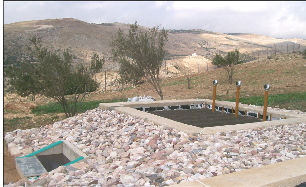
The recirculating vertical filter and flow splitter
